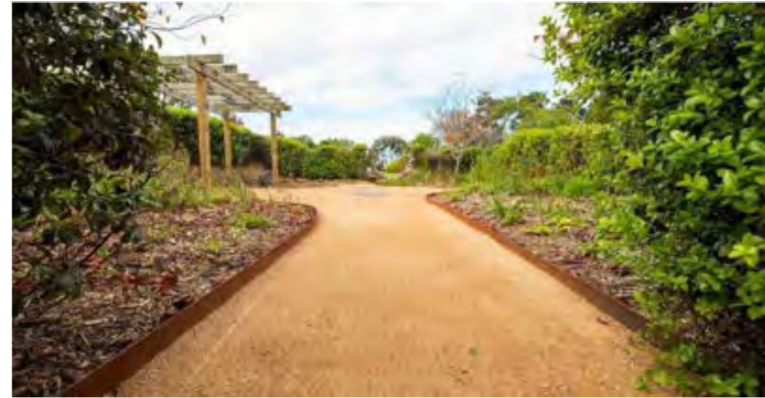
DG TO BE 3" THICK ORGANIC LOCK- GOLD, AVAILABLE AT GAIL MATERIALS. EPIC EDGING, AVAILABLE AT EPIC PLASTICS.
