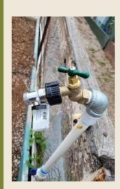
Many of the less expensive hoses feature aluminum hardware that, after time, will weld to the brass of the hose bib, causing the need to replace everything (the hose and the hose bib). Help minimize this by purchasing an adapter to attach to the hose bib before attaching your hose.
