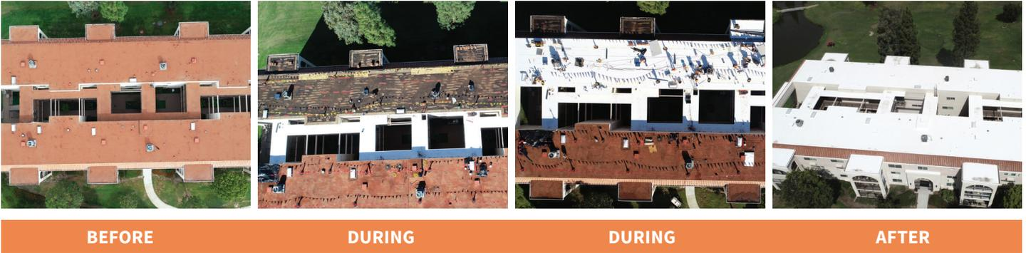
Built-up roofs are inspected 15 years after installation. Roofs determined to have reached the end of their serviceable life are scheduled to be replaced with a new PVC cool roof system. This year, 57 buildings are scheduled for roofing replacement. The program began late last month and is scheduled to be completed in October.
